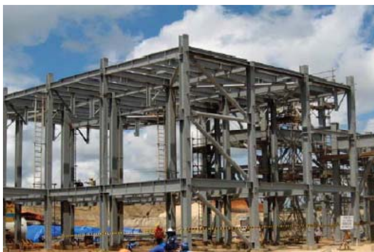
Figure 20 – Bayan plant under construction at the Tabang mine
