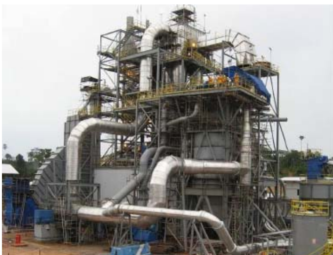
Figure 1 - Plant at the Tabang mine ready for commissioning
